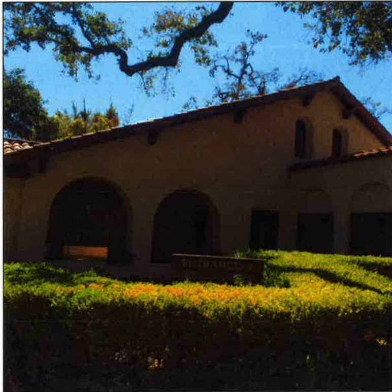
Plate 2. East end of façade displaying arched doors and windows, facing south.
