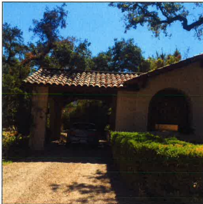
Plate 1. Arcaded porte-cochere at the east end of façade, facing south.
