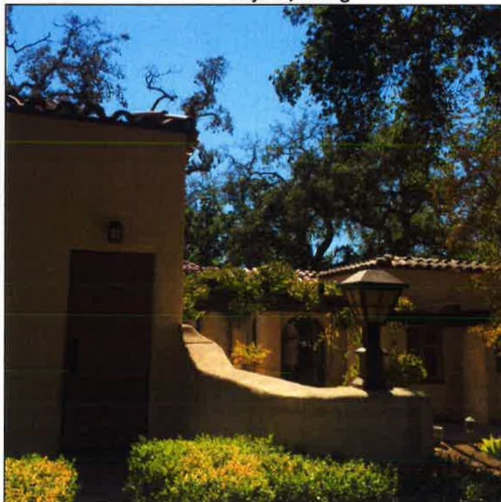
Plate 7. Façade – east of the City Hall courtyard entrance, facing south.
